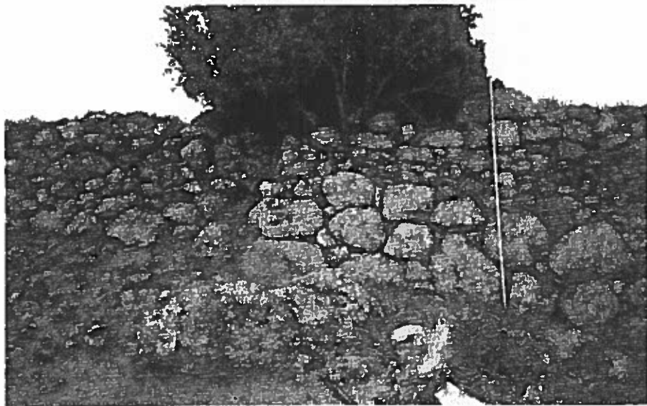
Plate 1. Geraki, acropolis wall at junction of Fields 30 and 26. Type 5c construction to left, built on ruins of earlier wall; gun emplacement to right of tree; masonry Types 1, 4, 5a-c
